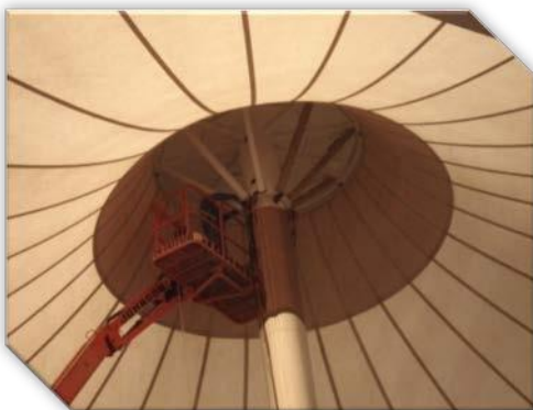
Fabric Installation
